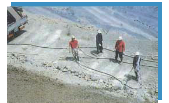
Spraying work in Kasama City, Ibaraki Prefecture
